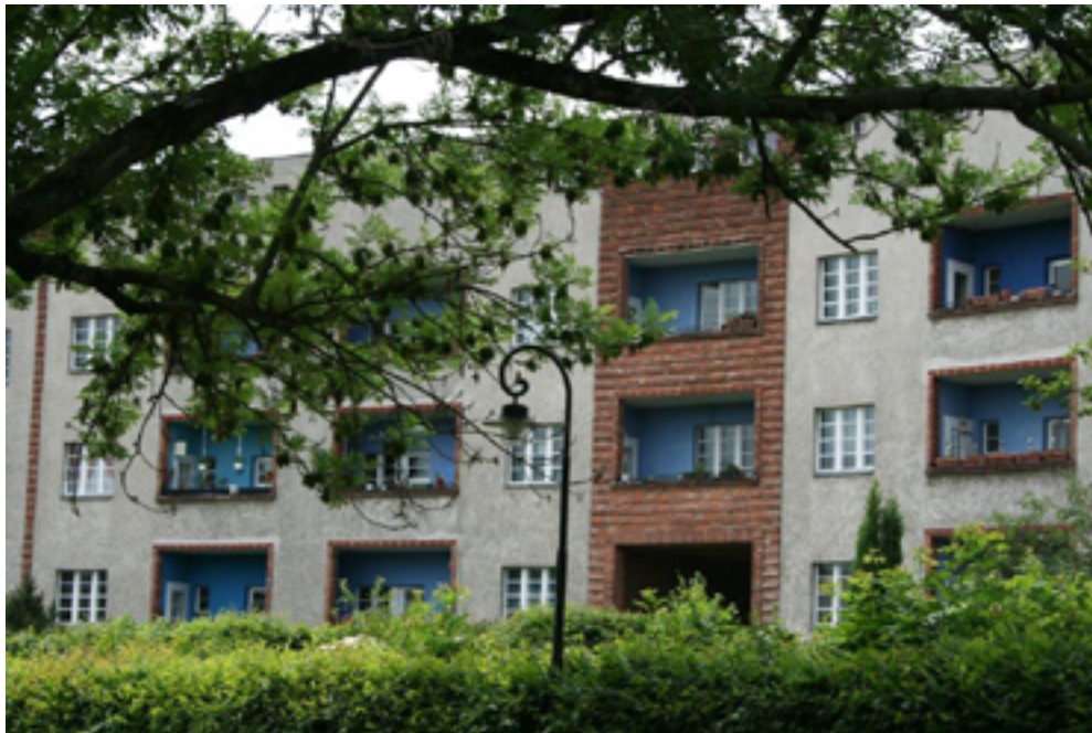
Using color to make buildings separate and distinct - a façade at the Horseshoe Estate
